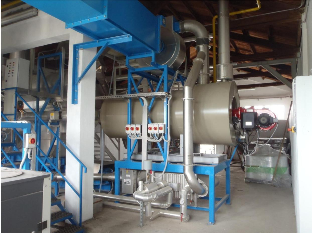
Supply air equipment including indirect burner (top), air chiller & reheater (bottom)
