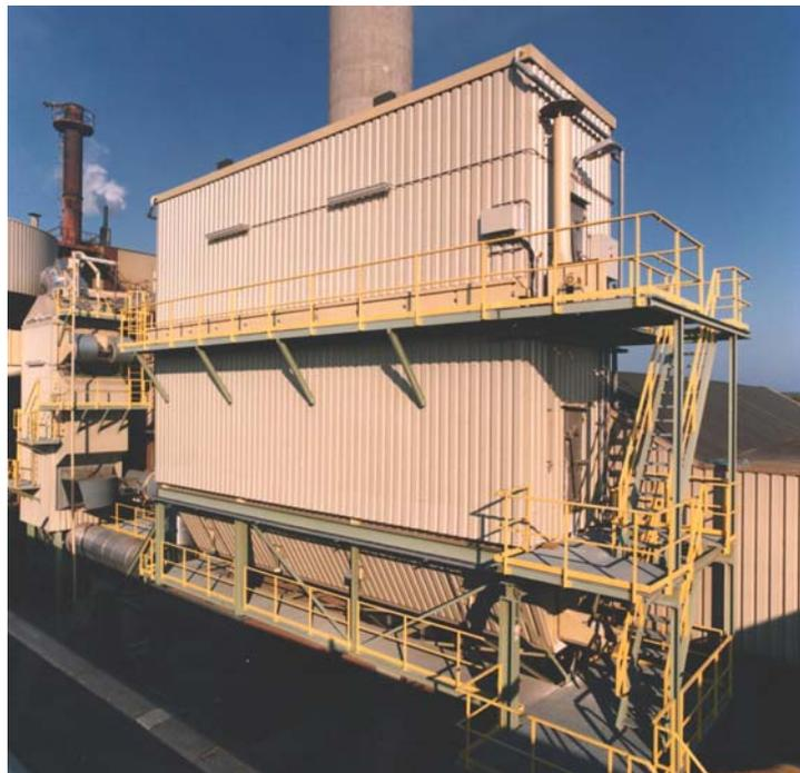
**JETBAG FILTER with automatic cleaned gas cooler**
