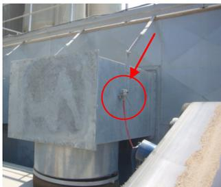
Image 2: Pressure Transmitter mounted to Air Outlet Ducting to baghouse.
